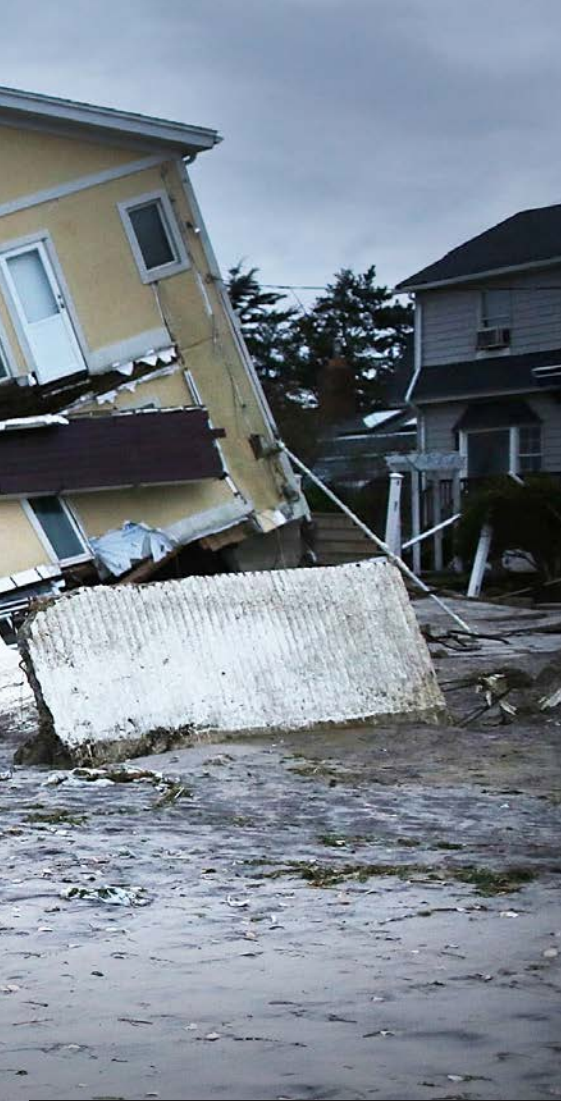
■ WASHED AWAY: Damage is viewed in the Rockaway neighborhood where a historic boardwalk was washed away during Hurricane Sandy in the Queens borough of New York City (Oct. 31, 2012).
