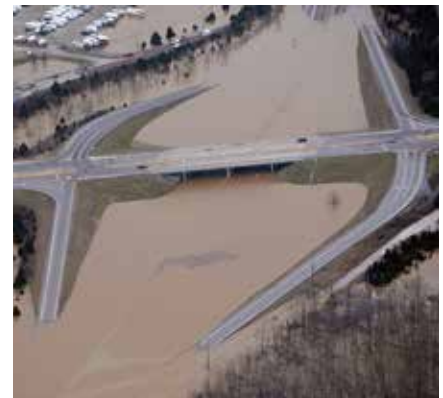
■ MAJOR FLOODING: Overflowing water from the Meremac River completely submerges Highway 141 in Arnold, Missouri, after the area received days of record rainfall (Dec. 31, 2015).
