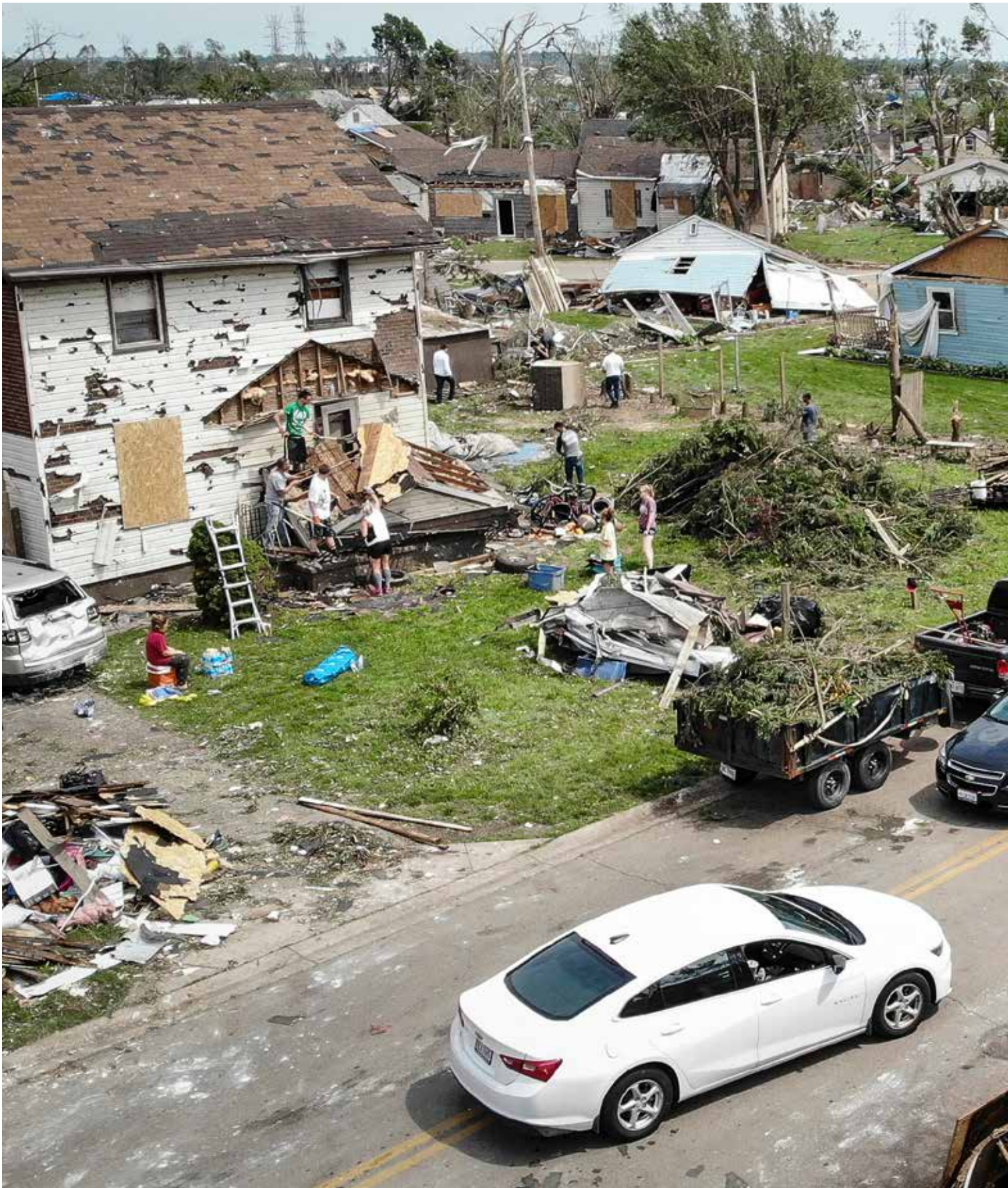
Residents clean up a tornado-damaged neighborhood in Dayton, Ohio (May 29, 2019). Photo: AP/John Minchillo
