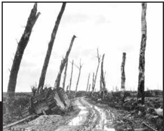
Dec. 19, 1918: What is left of a street corner in Poelcapelle, Belgium.
