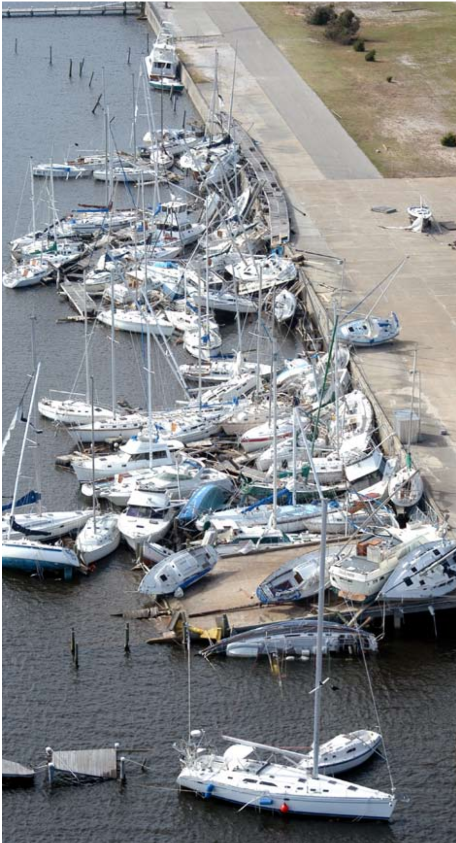
■ IVAN'S AFTERMATH: In Florida, Hurricane Ivan sunk and stacked numerous boats at Bayou Grande Marina onboard Naval Air Station Pensacola. Navy officials reported that nearly 90% of the buildings on the base suffered significant damage (Sept. 22, 2004).
