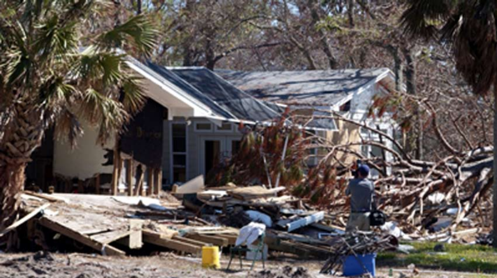
■ ONE OF MANY HOMES LOST: Thousands of Pensacola area residents were displaced from their homes, which were damaged by Hurricane Ivan (Oct. 13, 2004).
