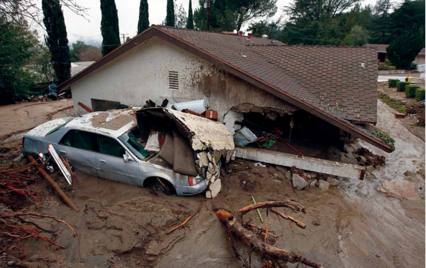
■ INUNDATED: A mudflow carrying debris damages a house after heavy rains in La Canada Flintridge, California (Feb. 6, 2010). PHOTO: DAVID MCNEU/AFP/GETTY IMAGES
