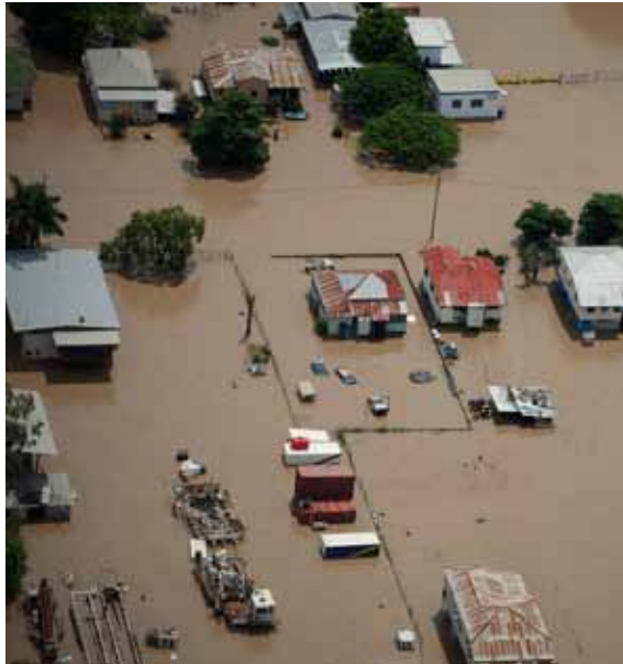
■ INUNDATED: An aerial photo shows the flooded Depot Hill area south of Rockhampton, Queensland (Jan. 6, 2011).
