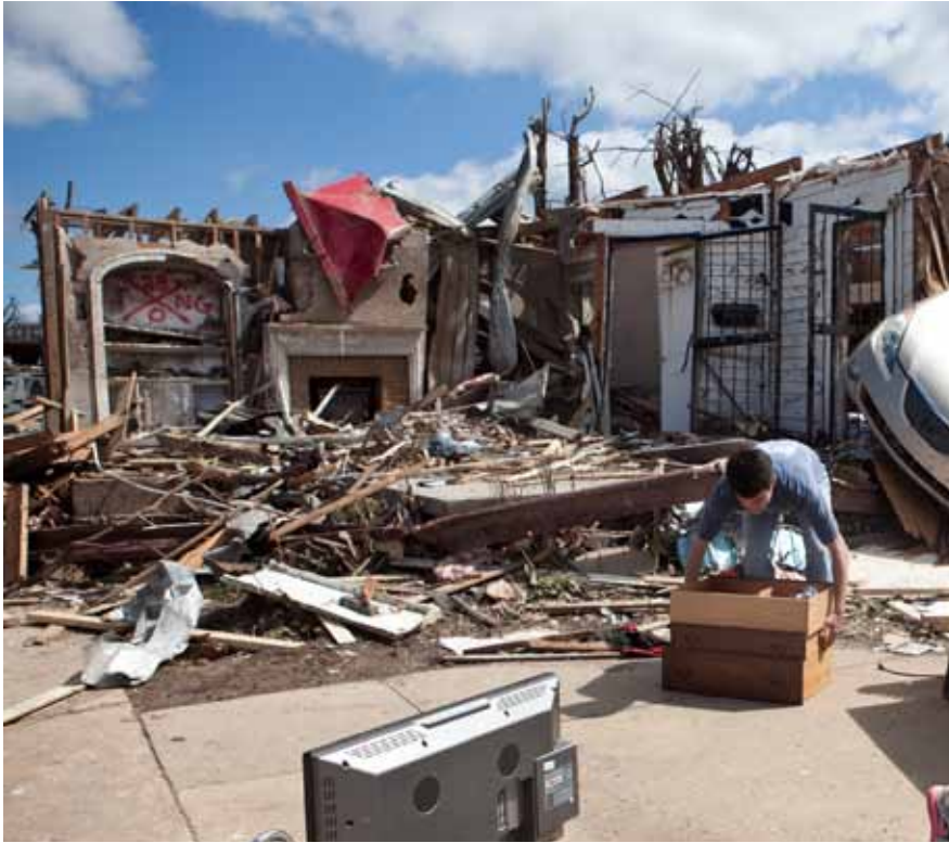
■ DESTRUCTIVE PATH: In the aftermath of a severe tornado, debris from destroyed homes is strewn across lawns in Tuscaloosa, Alabama (April 28, 2011).
