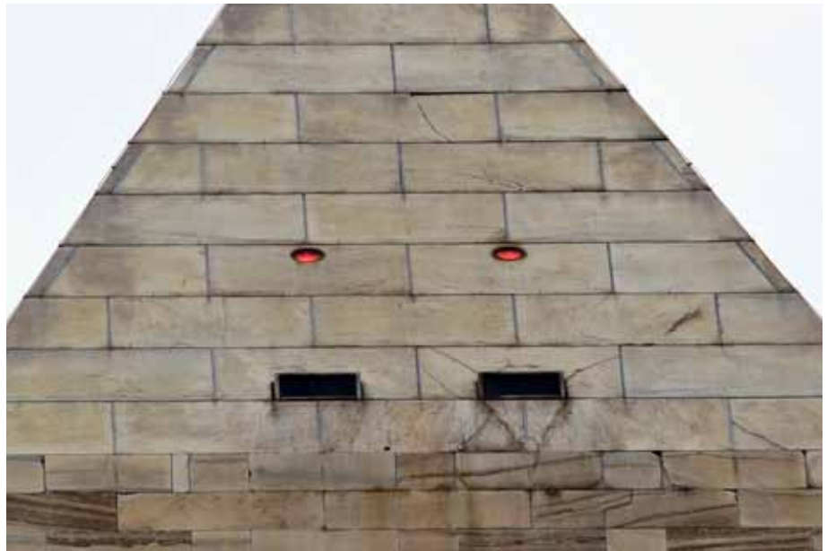
■ DAMAGED: A crack shows on the top west face of the Washington Monument after an earthquake struck the region (Aug. 25, 2011).
